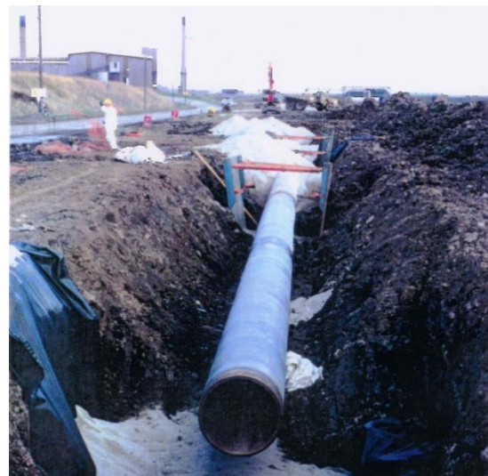
Construction Images of the 36" pipeline routing through South Tees industrial sites
