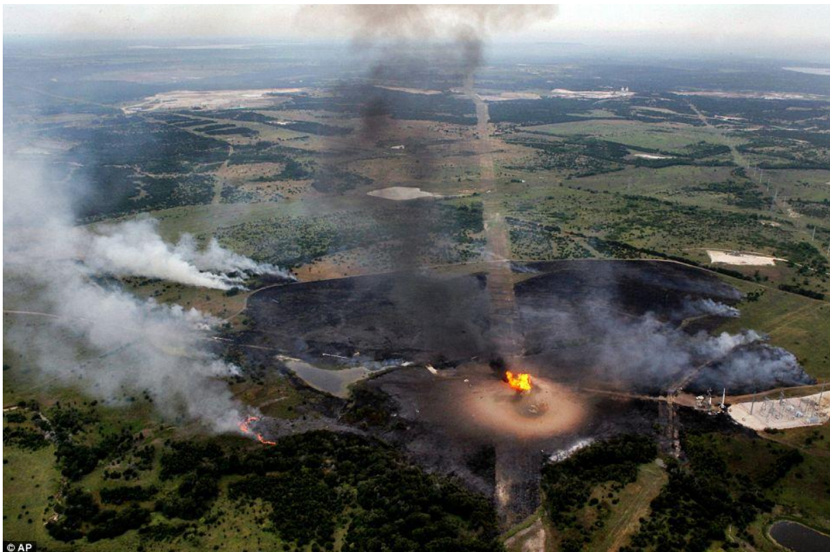
36" Gas Pipeline Explosion, North Texas June 7, 2010
