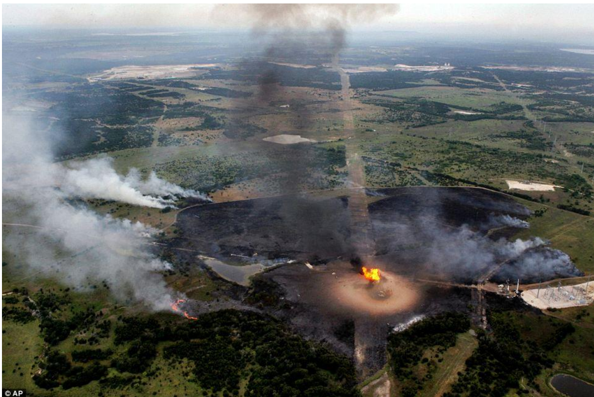
36" Gas Pipeline Explosion, North Texas June 7, 2010
